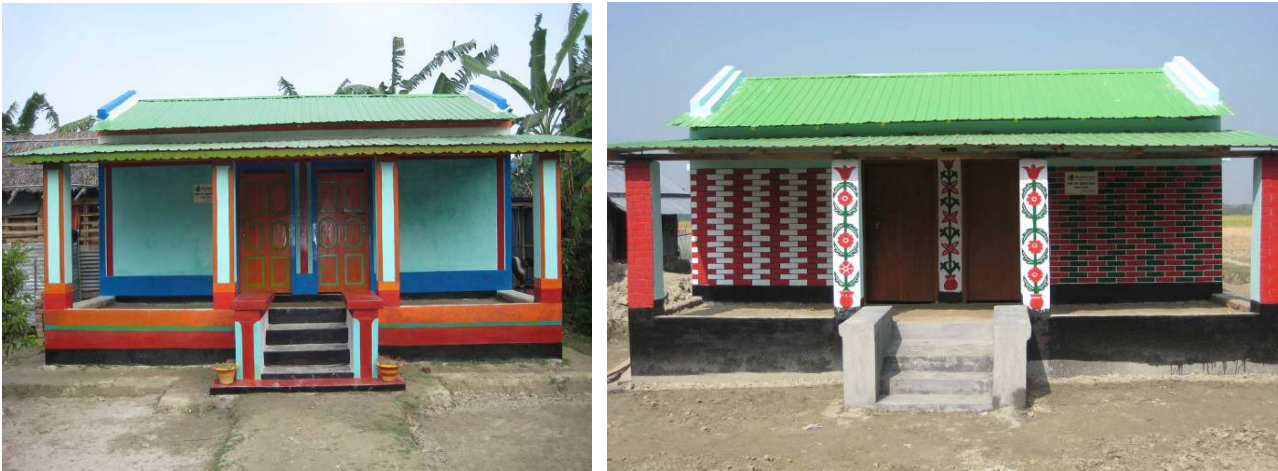
'Two Part' roofing but with different painting designs as per beneficiary's individual preferences.
