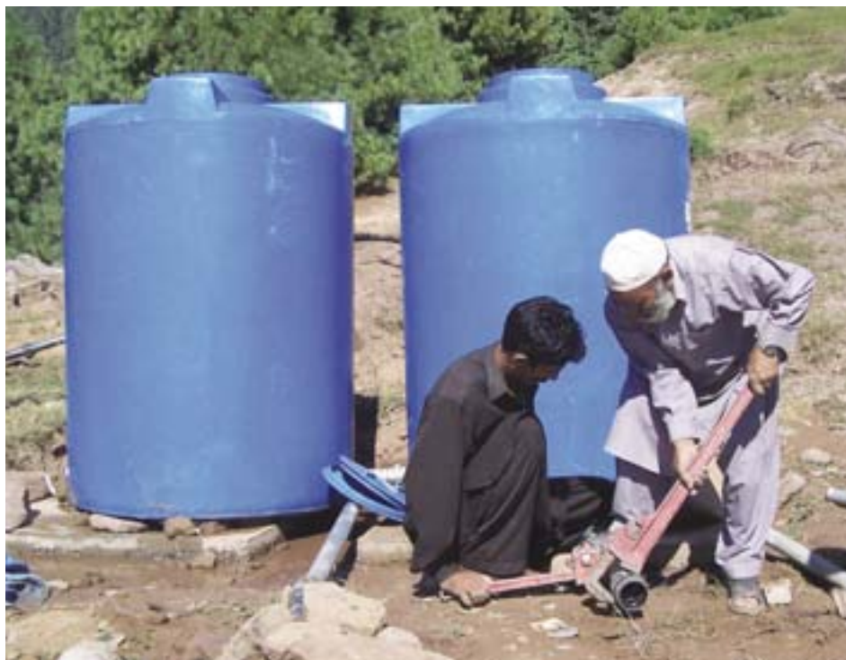
Installing Dara water system, Bagh District.
