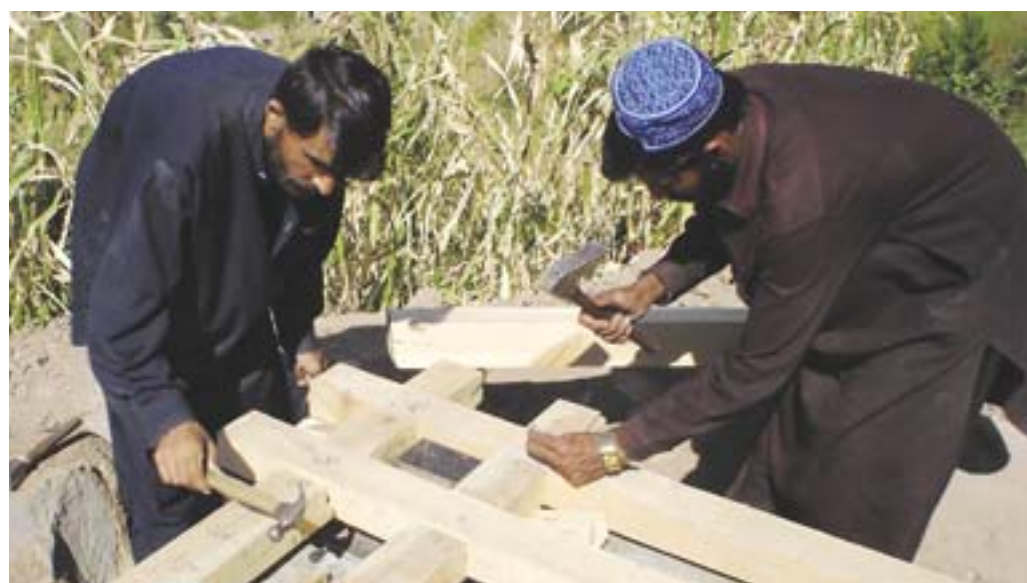
Construction of earthquake-resistant 'demo' house.
