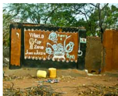
One of the house that was destroyed in Hagadera
